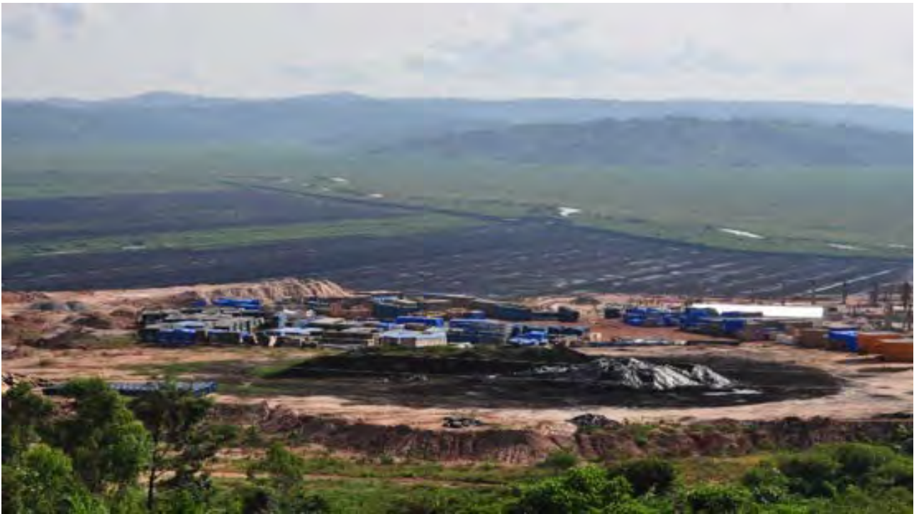
Figure 3.14. Peat-powered electricity plant in Gisagara, Rwanda. Photo: Hans Joosten
